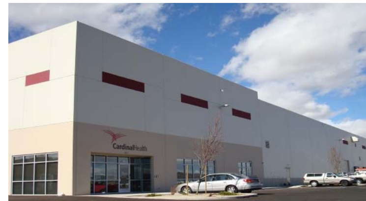
Reno, NV, Distribution Center
